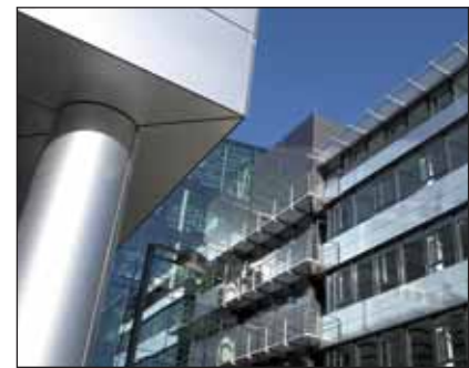
In 2005, 35 million euros were invested in the 16,000 m 2 construction
